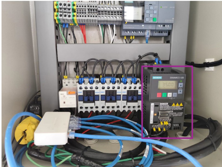
Figure 9. Centrifugal fan speed controller
